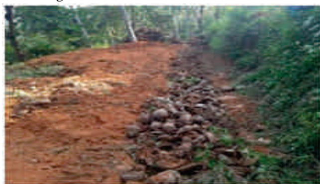
Fig. 52. Trench filled with coconut husk
